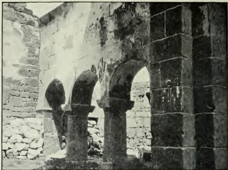
FIG. 306.—Sivri Hissar, arcade between nave and aisle.
